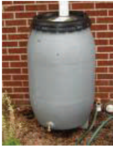
Water flowing into a homemade rain barrel from a downspout.
